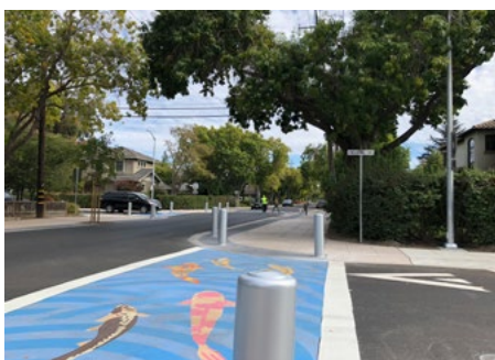
Asphalt raised intersection in Palo Alto, CA
